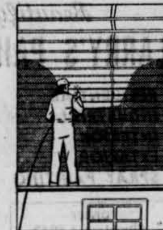
Dirty Black Concrete
