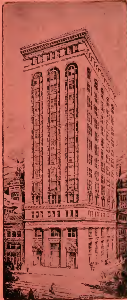
METROPOLIS BANK BUILDING
