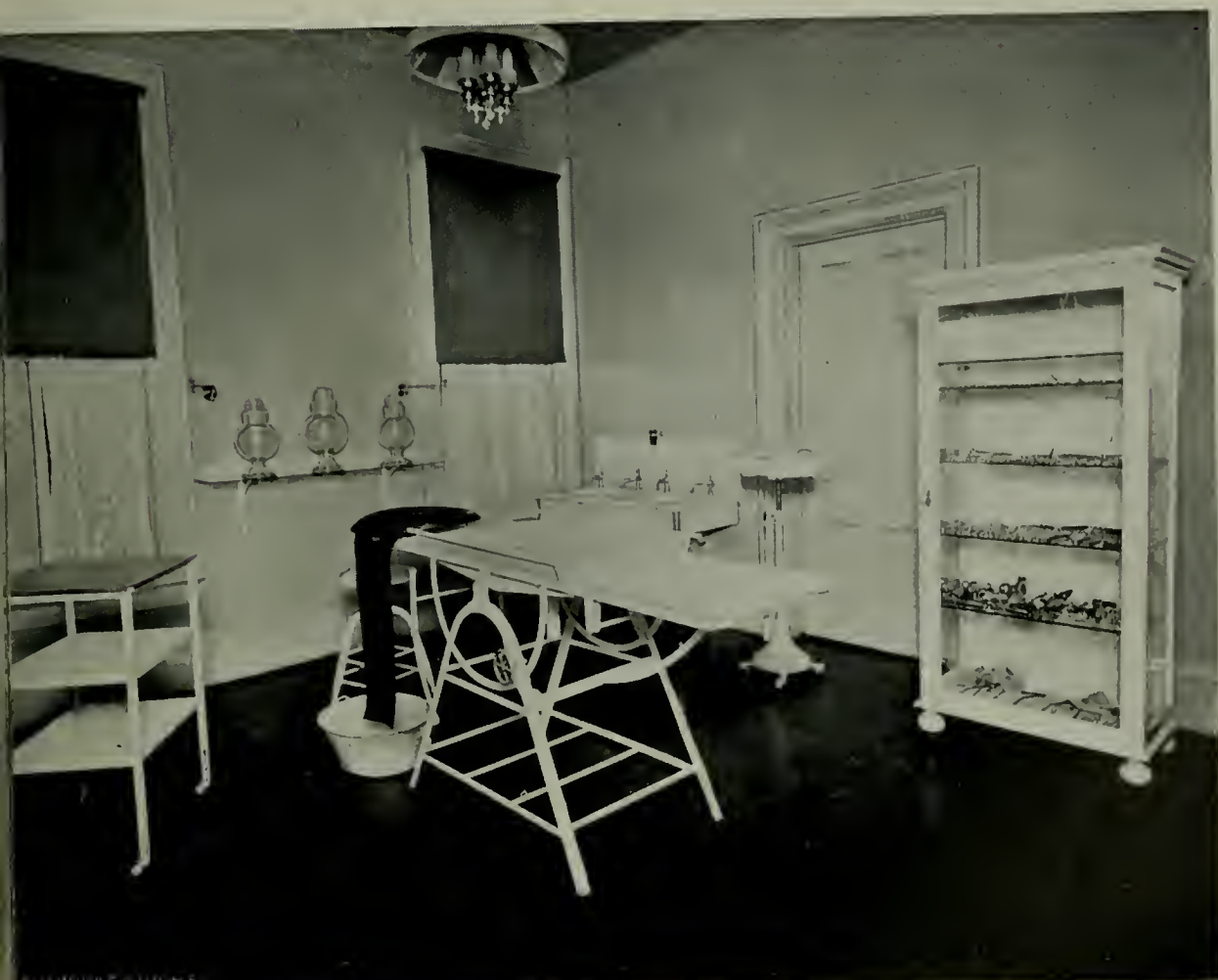
GENERAL OPERATING ROOM, ENAMEL AND GLASS FINISH.
