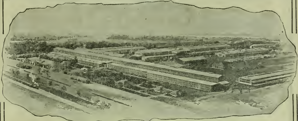
Works: Sunnyvale, California
