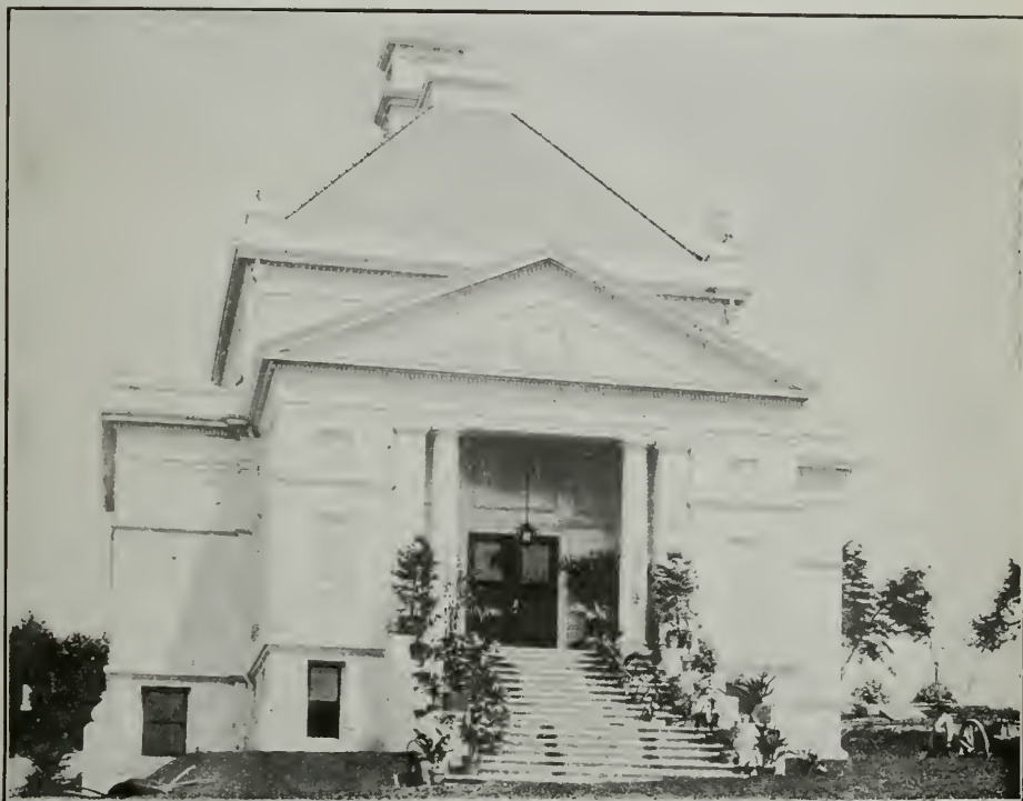
Front view of the Crematorium, showing entrance to the Chapel.
