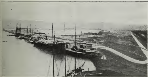
THE PARR TERMINAL ON OAKLAND'S WATER-FRONT
