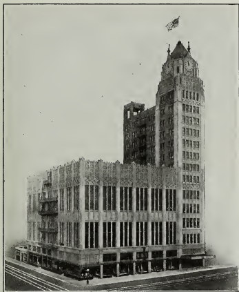
ELKS CLUB BUILDING, OAKLAND
