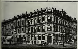
OAKLAND BANK OF SAVINGS Northeast corner, Twelfth and Broadway
