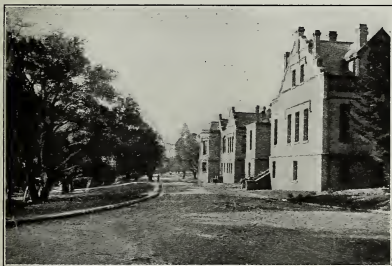
SOUTH FRONT, CHEMISTRY BUILDING, 1895
