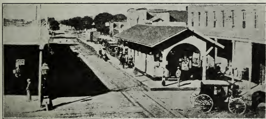
OAKLAND'S FIRST RAILROAD STATION AT SEVENTH AND BROADWAY On the left is the first gas light erected in Oakland, first spreading its gleams of light over that corner on December 31, 1866
