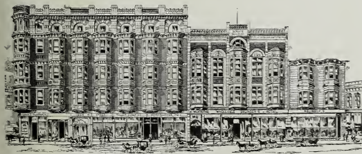
WASHINGTON STREET, WEST SIDE, FROM TENTH TO ELEVENTH STREETS, OAKLAND, 1896 Hotel Crellin on left; Salinger's Department Store on right
